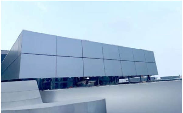
Beijing Guangqu Jinmao Palace uses the grey photovoltaic wall product and the hidden-framed photovoltaic wall system, with an installed capacity of 3.4 kW
