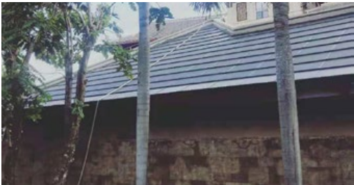
Jinmao Ritz-Carlton Sanya uses the grey photovoltaic tile product, REC batteries, and our self-developed photovoltaic tile system, with an installed capacity of 4.6 kW
