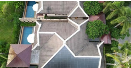
Jinmao Ritz-Carlton Sanya uses the grey photovoltaic tile product, REC batteries, and our self-developed photovoltaic tile system, with an installed capacity of 4.6 kW
