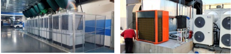
Air-source heat pump water heaters
